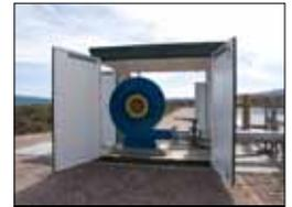
*Low pressure, low energy fan blowers require little maintenance and only run when required by loading.*
