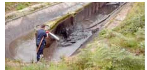
*Sludge and peak flows from the existing ditch are diverted to the Aero-Fac® Sludge Digestion System.*
