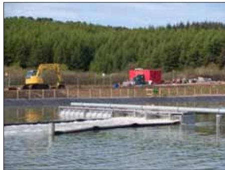
*Unlike conventional diffused air systems, the 100% stainless steel diffused air system has no moving parts, and requires no routine servicing or maintenance.*
