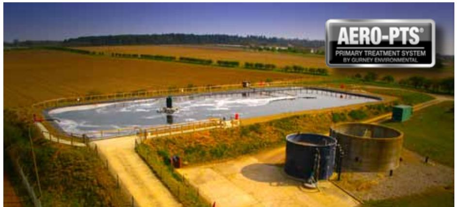
*The Aero-Fac PTS in use for 7 years at East Harling, Norfolk. The PTS system provides primary treatment in front of conventional filters, buffering storm surges and handling all solids.*
