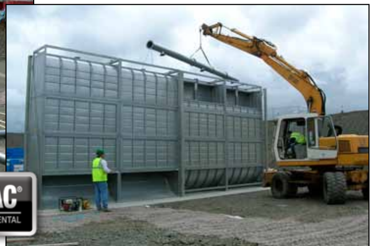
The Aero-Fac® plant for Scottish Water was put into service at Tobermory on the Isle of Mull in 2007. The simple installation of aeration modules was easily carried out over the course of a few days.
