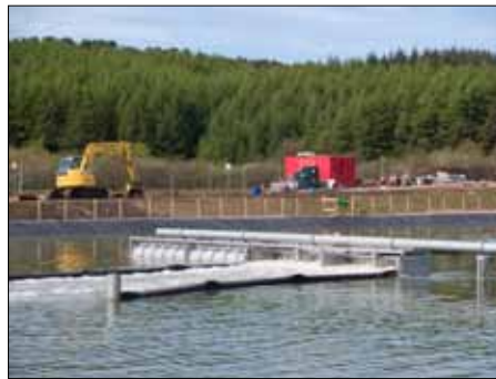
Unlike conventional diffused air systems, the 100% stainless steel diffused air system has no moving parts, and requires no routine servicing or maintenance.
