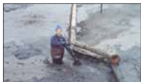
Four decades of intensive research into lagoon design and sludge digestion provides the basis for Gurney Environmental's unique designs and technologies.
