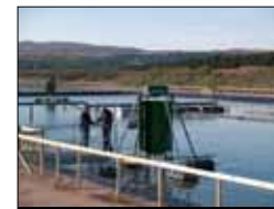
Unique wind powered aeration/optimisation units keep annual energy costs low.
