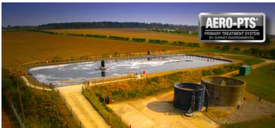
The Aero-Fac PTS in use for 7 years at East Harling, Norfolk. The PTS system provides primary treatment in front of conventional filters, buffering storm surges and handling all solids.
