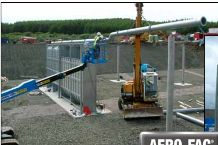
The Aero-Fac® plant for Scottish Water was put into service at Tobermory on the Isle of Mull in 2007. The simple installation of aeration modules was easily carried out over the course of a few days.
