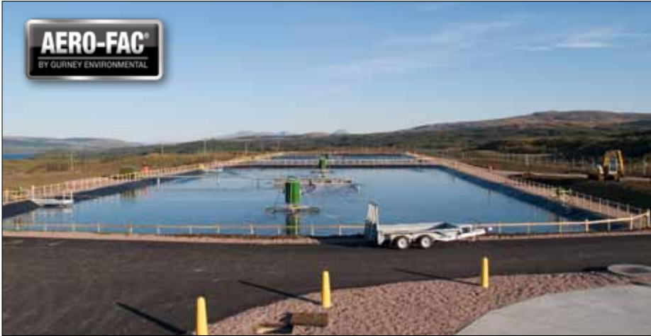
The Aero-Fac® WWTP at Tobermory, Scotland was commissioned for Scottish Water in May 2007. The system features no sludge, low energy, low manpower and maintenance — all important issues for an island wwtp.
